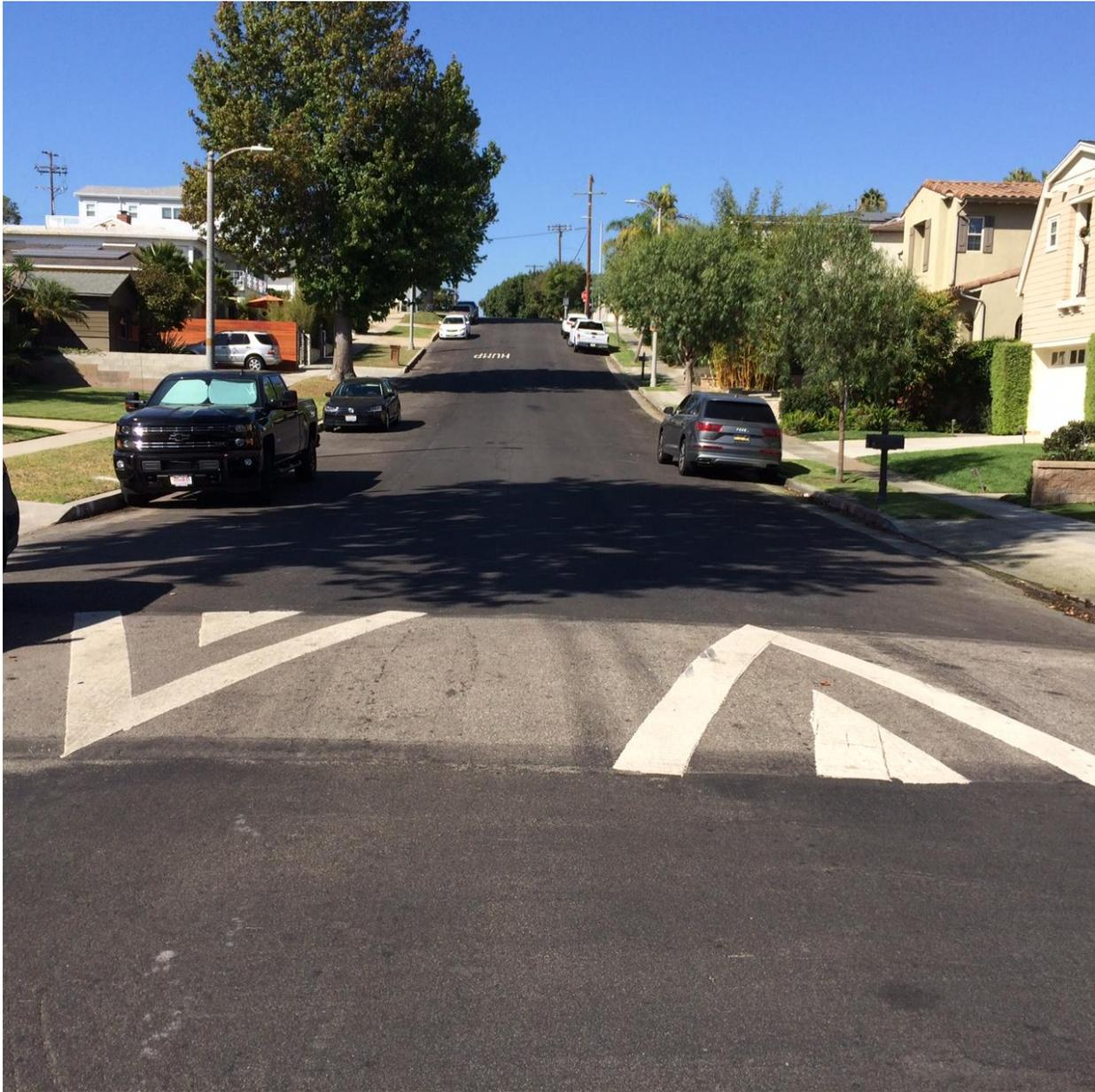
[This speed hump is located on the section of the block where the grade is less than 7% but as far up the hill as possible.]
