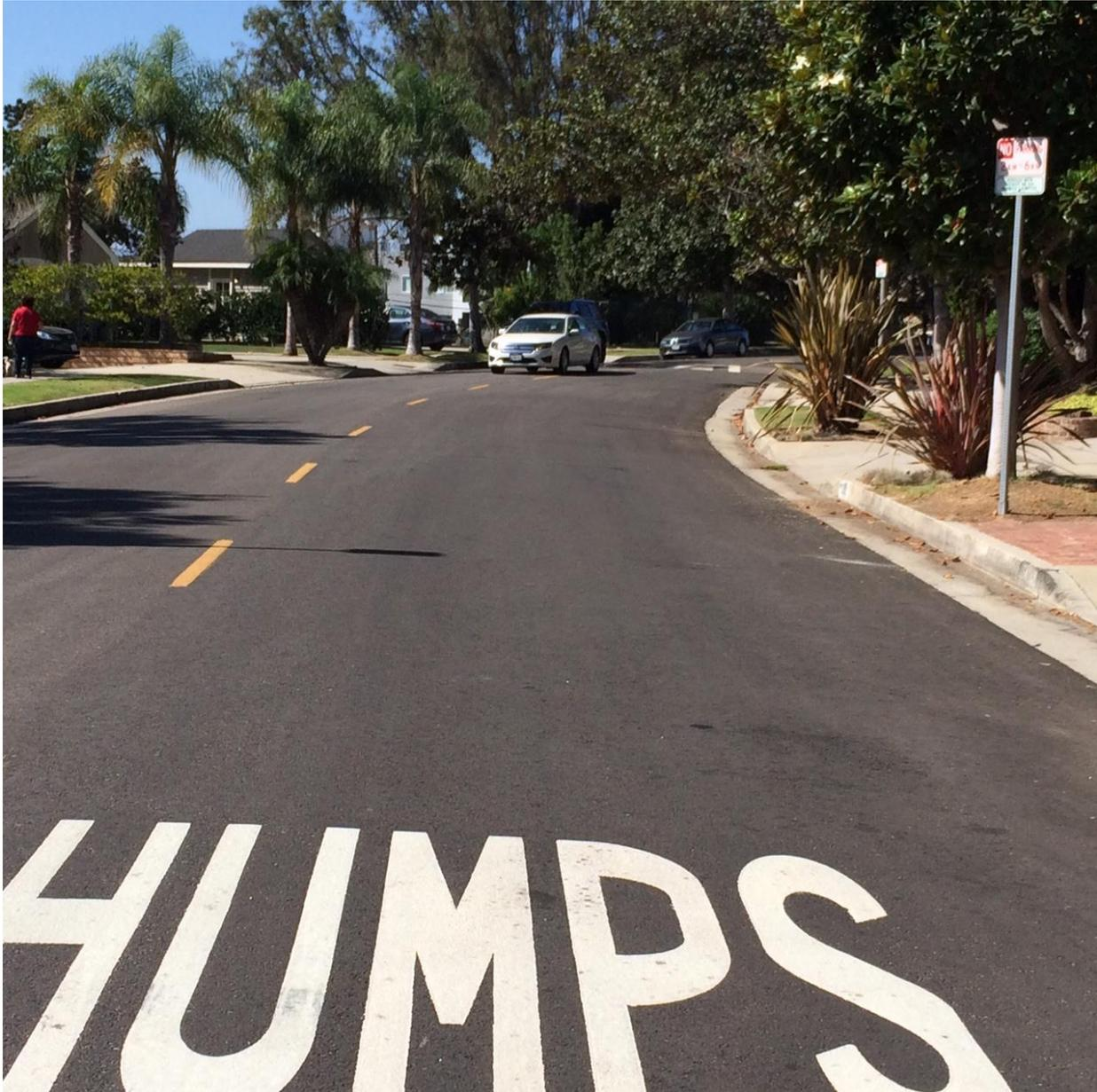
[The speed hump at the top of the picture is visible from the "HUMPS" marking at approximately 200 feet away]
